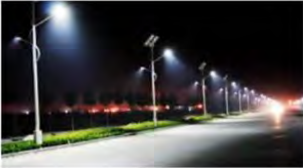
Solar Street Lighting
